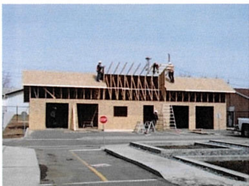
Jeep Storage Garage construction
